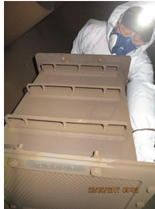
Inspection of field test catalyst device in exhaust manifold
