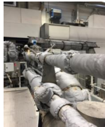
Mini SCR system for urea mixing/evaporator study
