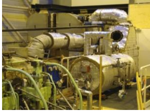
High Pressure Boiler installed on 4T50ME-X
